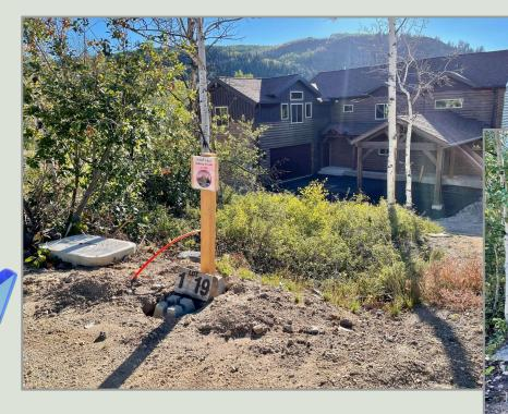
There is typically a 30"W x 48"L x 24"D vault that serves 2-to-4 homes. The orange tube is for a 1" line with pull tape.
