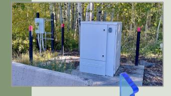
Primary Fiber Network and Power Node with Backup. There is typically a 30"W x 48"L x 24"D vault that serves 2-to-4 homes. The orange tube is for a 1" line with pull tape.
