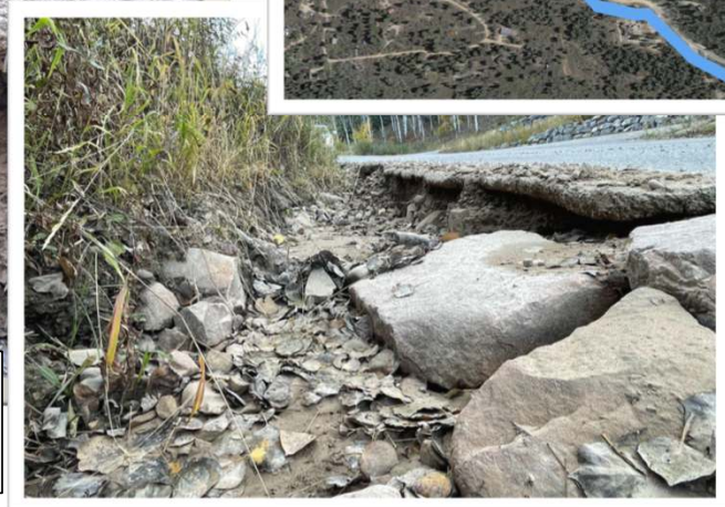
This is a section of TGC Road along the western edge above Hillcrest that has nothing protecting it to a depth of 10-to-12-inches.
