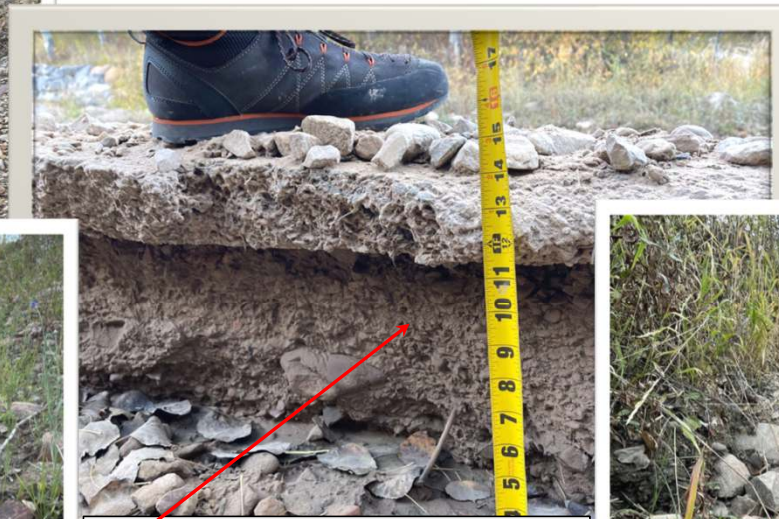
This is a section of TGC Road along the western edge above Hillcrest that has nothing protecting it to a depth of 10-to-12-inches.
