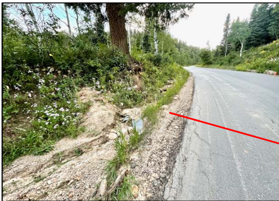
Buried Culvert underneath TGC Road is unable to move water
